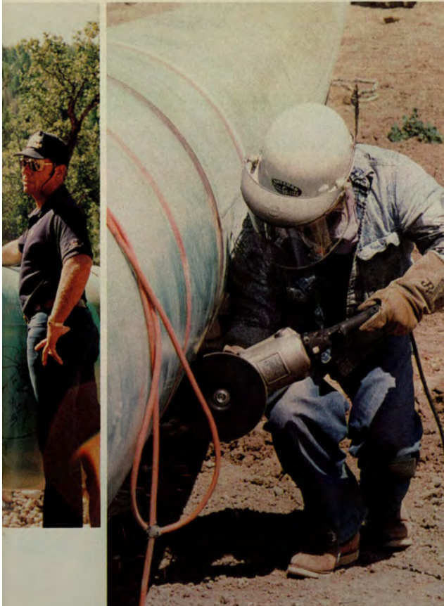
A helper on the pipeline performs grinding work.
