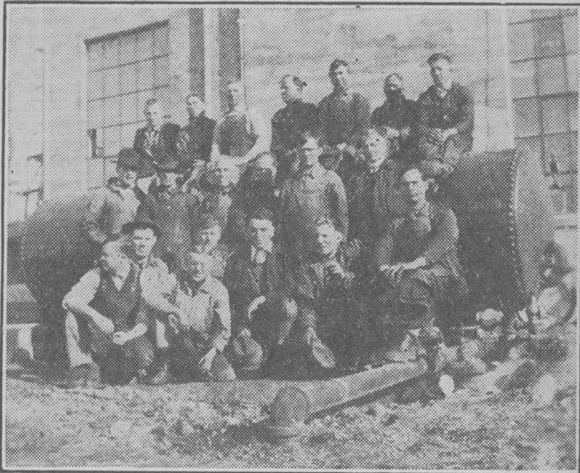
The Steamfitters of Local 342 on the One Million Dollar Sherwin & Williams Paint Manufacturing Plant Located at Emoryville, Oakland. Reading from left to right (upper)—Bro. Shaw, President of Local 342; Bro. Hendrix, Bro. Reeder, Bro. Kaufman, Bro. Woods, Bro. Taber, Bro. Helper, Bro. Kingsley, Bro. Anderson, Bro. Hartley, Bro. McCaabe, Bro. Davis, Bro. Mooney, Bro. Gannon, Bro. O'Connor, Bro. Dinsmore, Bro. May, Bro. Edwards, in Charge of Construction; Bro. Marsh and Bro. Winton.
